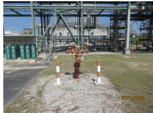
Water Monitor with Remote
