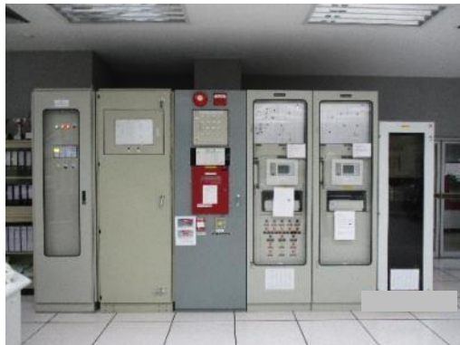
Master Fire Alarm Control Panel
