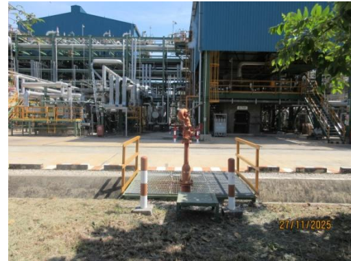
Water Hydrant with Monitor
