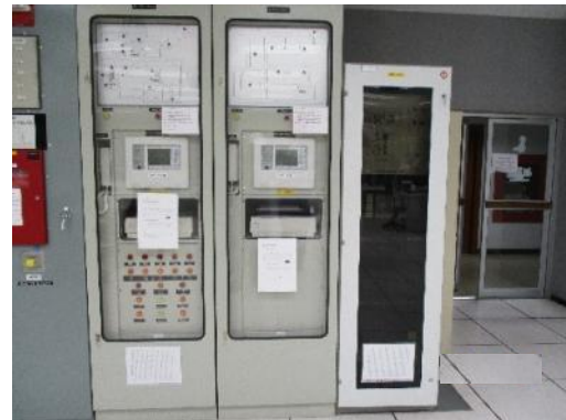
Slave Fire Alarm Panel
